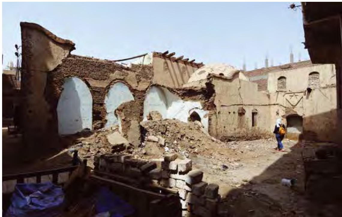
The façade of the Abd el-Rassoul House. Photo: Zs. Vasáros, 2019.
